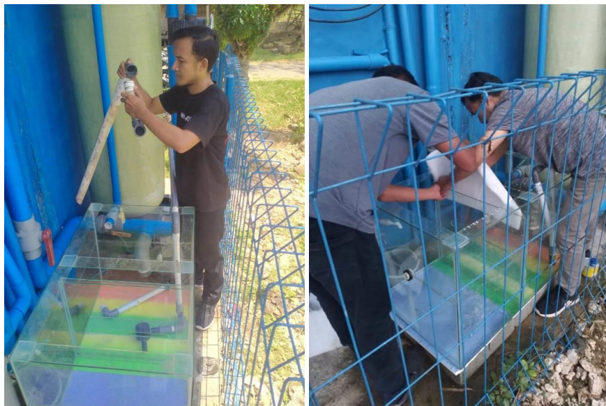
Gambar 2. Proses pemasangan filter MBG
